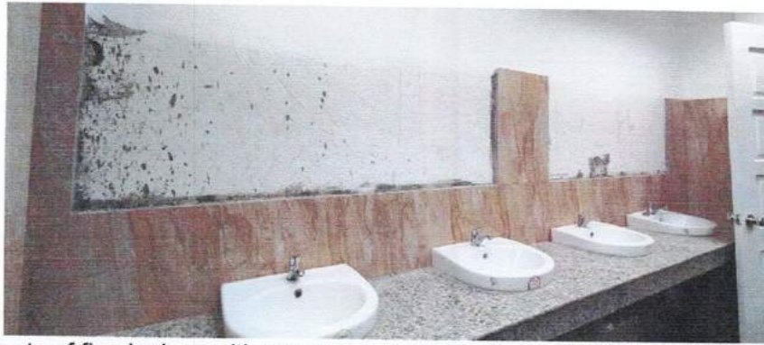
Two (2) sets of fixed mirror with approximate dimensions: (Verify Actual Measurement) Length = 1.70m, Height = 0.60m (Left); Length = 1.50m, Height = 0.60m (Right)
