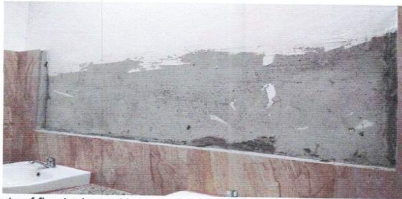
Two (2) sets of fixed mirror with approximate dimensions: (Verify Actual Measurement) Length = 1.55m, Height = 0.60m
