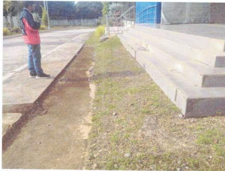
Approximate Length = 8.70m ( Verify Actual Measurement )
