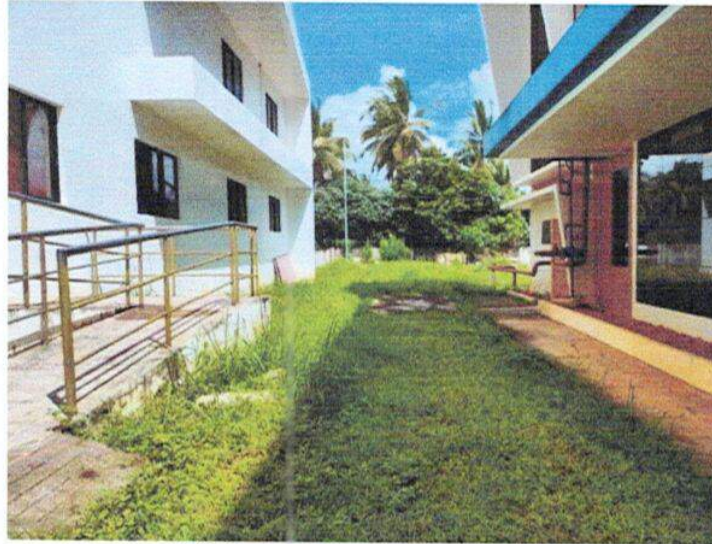
(a) Actual site condition of the area
