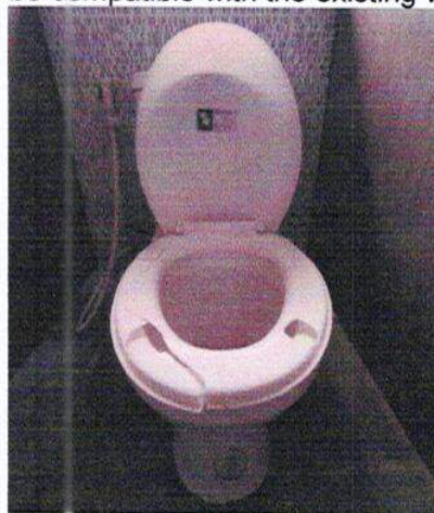
Damaged Water Closet Cover
