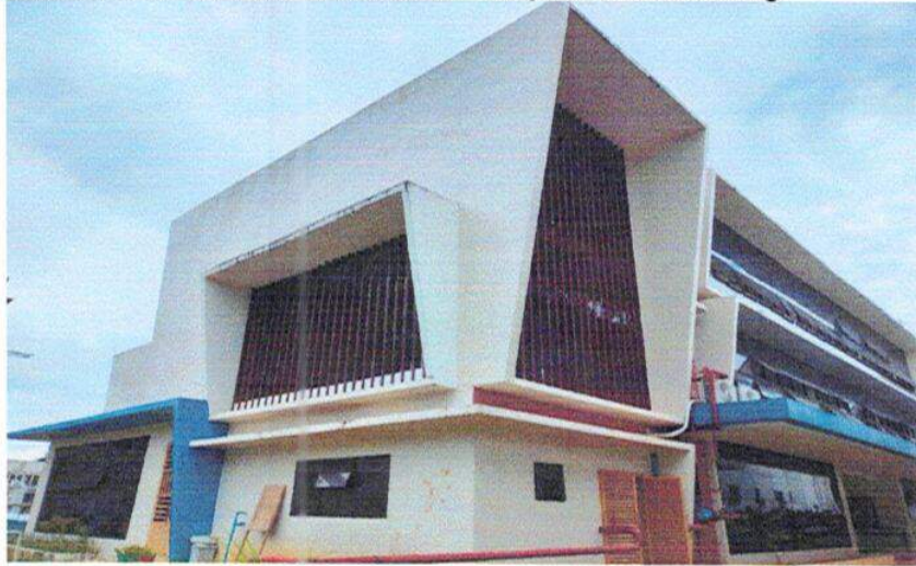
Peeled-off Paints on Vertical Slats
