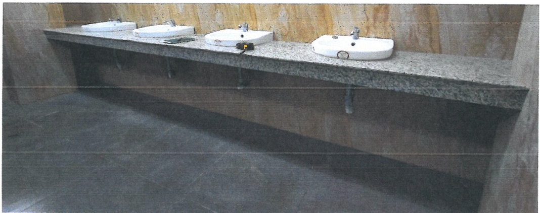
Two (2) sets of cabinetry with approximate dimensions: (Verify for Actual) Length = 3.70m, Height = 0.75m, Width = 0.50m
