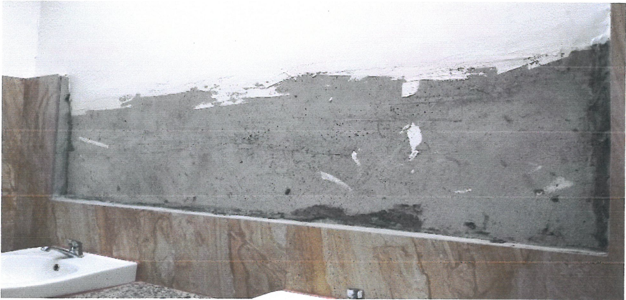
Two (2) sets of fixed mirror with approximate dimensions: (Verify for Actual at Men's Toilet) Length = 1.55m, Height = 0.60m
