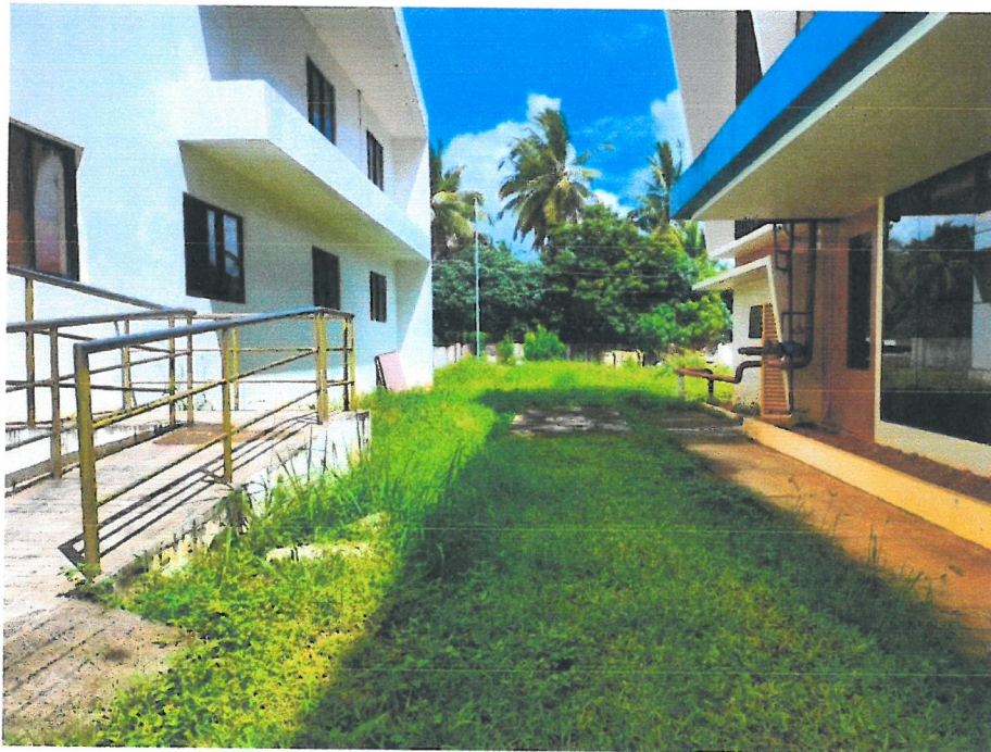
(a) Actual site condition of the area
