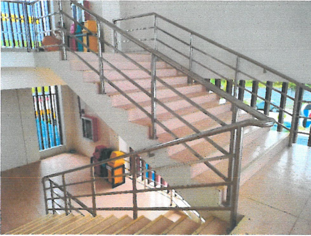
(a.1.) Stainless Steel Railings
