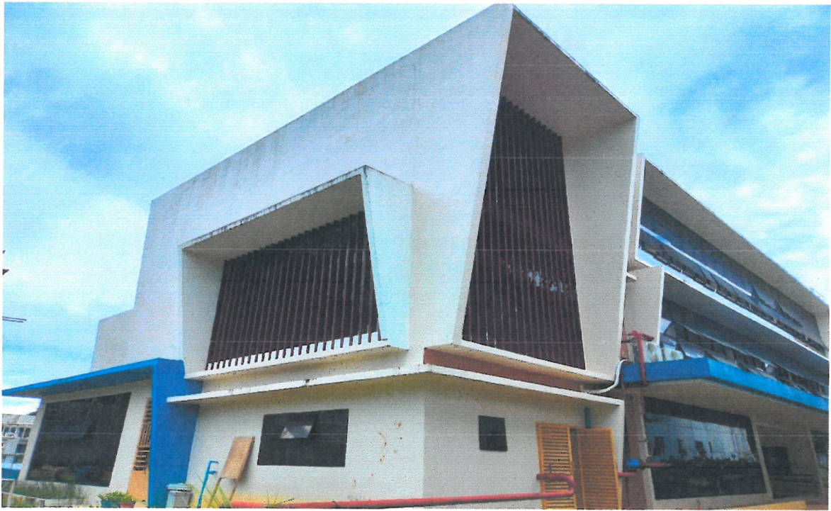
(b.1.) Peeled-off Paints on Vertical Slats
